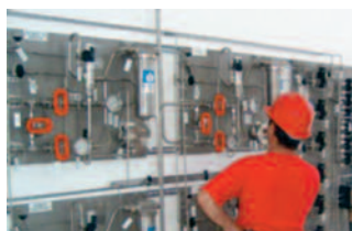
Fast loop panel installation
